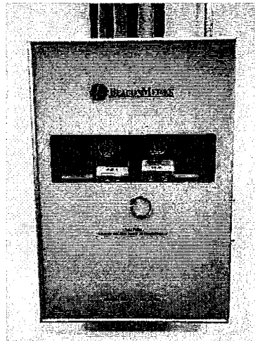
Oxygen valve panel
