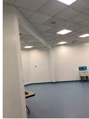
Photo 19: POC Testing Room – Framed Opening with New Floor and Sink
