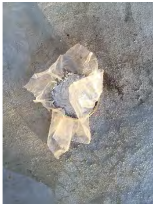
Photo 67: Oxygen Distribution System – Storm Water Drains Plugged at Bulk Storage Location
