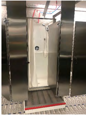
Photo 24: Northeast Women's Restroom – Toilet Stall Converted into Shower Stall
