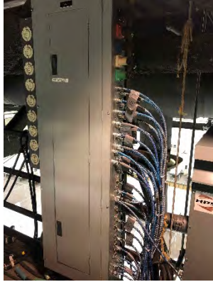
Photo 41: Emergency Power Supply Tying into Existing System at Catwalk
