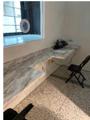
Photo 17: Outpatient Pharmacy – Counter Installed with Notch to Allow Use of Pass-Through Drawer for Rx Distribution
