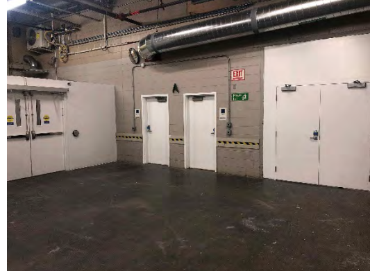
Photo 15: Inpatient Pharmacy and Central Clean Storage – Doors with Trilogy Locks Added
