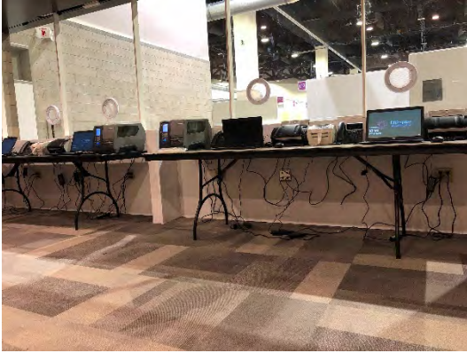
Photo 18: Registration – Half-Wall with Plexiglass Windows and Talk-Through Portals Installed
