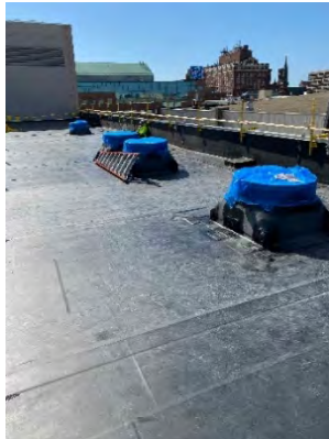
Photo 27: Penetrations at Roof for Exhaust Ducts
