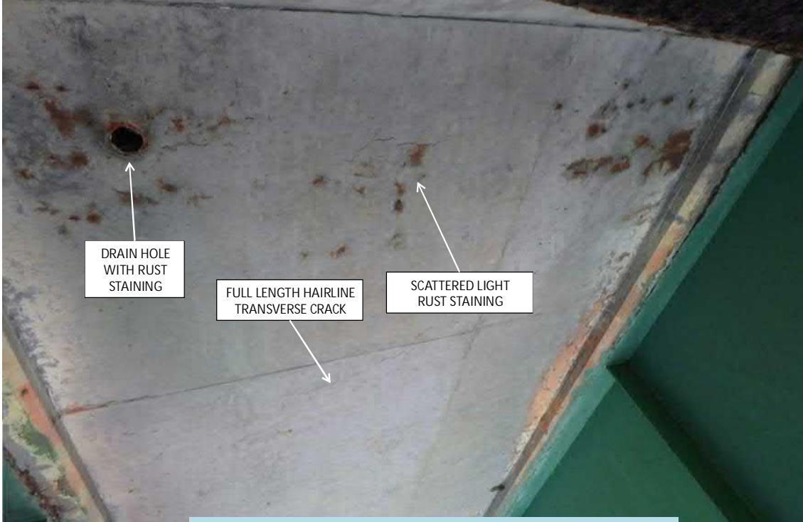
BRIDGE #067301 UNDERSIDE IN BAY 'F' –AT PIER 1 IN SPAN 1 (LOOKING SOUTH) 8/2/2018
