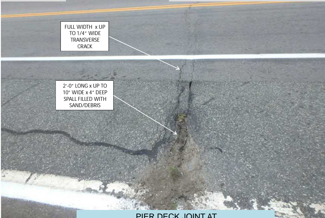
PIER DECK JOINT AT BRIDGE #067301 PIER 1 EAST SHOULDER (LOOKING WEST) 8/2/2018
