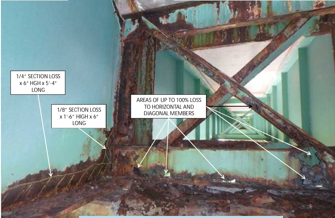
GIRDER 'F' – WEST FACE BRIDGE #067301 AT PIER 1 IN SPAN 2 (LOOKING NORTHEAST ) 8/2/2018
