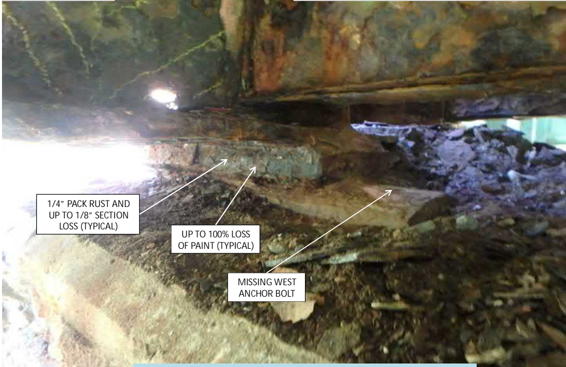
BEARING 'G' – AT PIER 1 IN SPAN 2 (LOOKING EAST)
