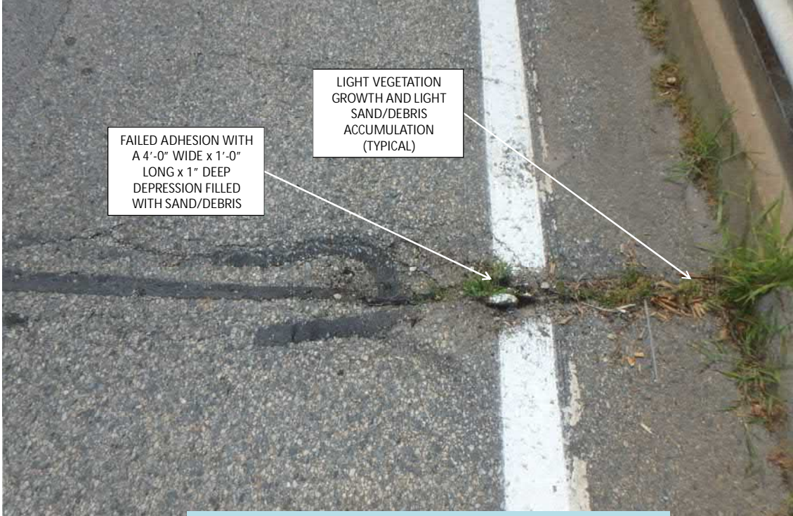
PIER DECK JOINT AT BRIDGE #067301 PIER 1 WEST SHOULDER (LOOKING SOUTH) 8/2/2018
