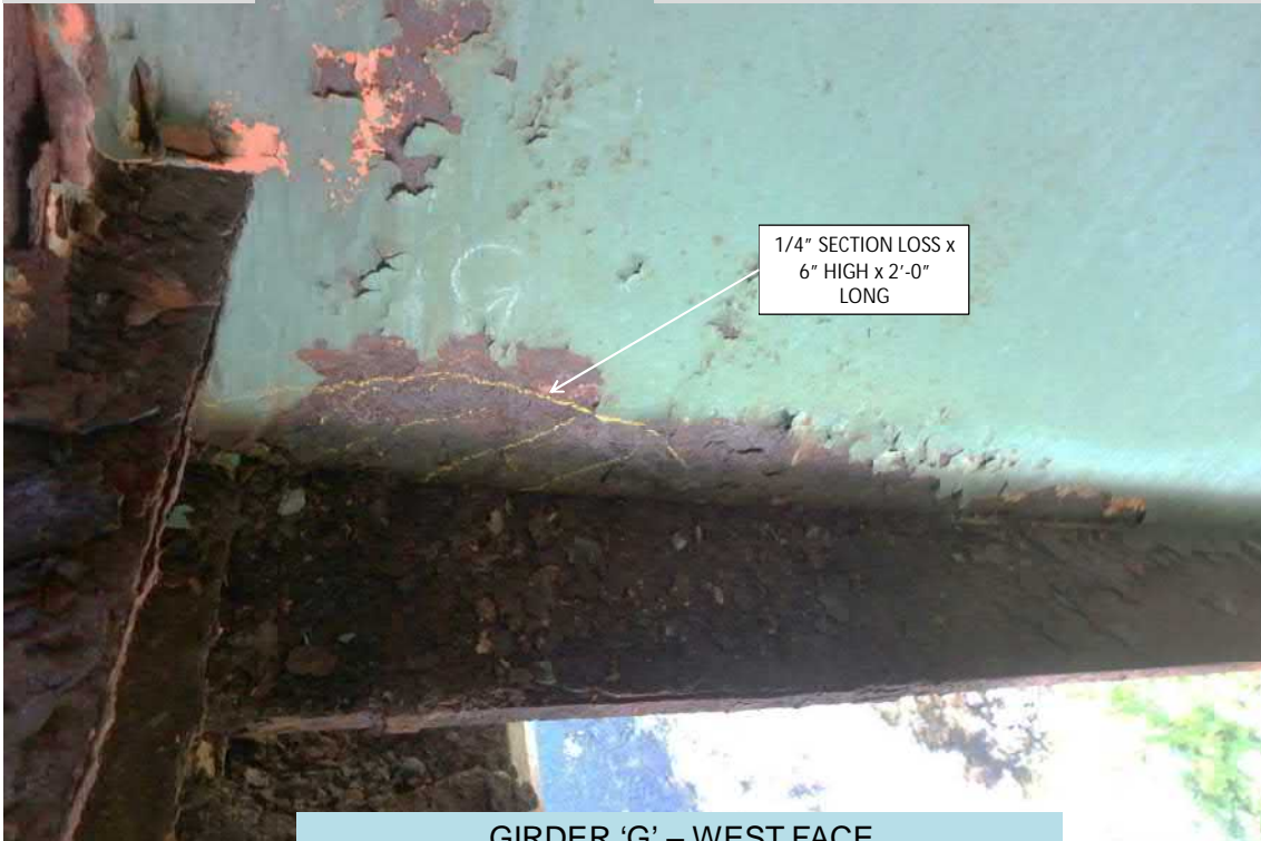
BRIDGE #067301 GIRDER 'G' – WEST FACE AT PIER 1 IN SPAN 1 (LOOKING EAST) 8/2/2018
