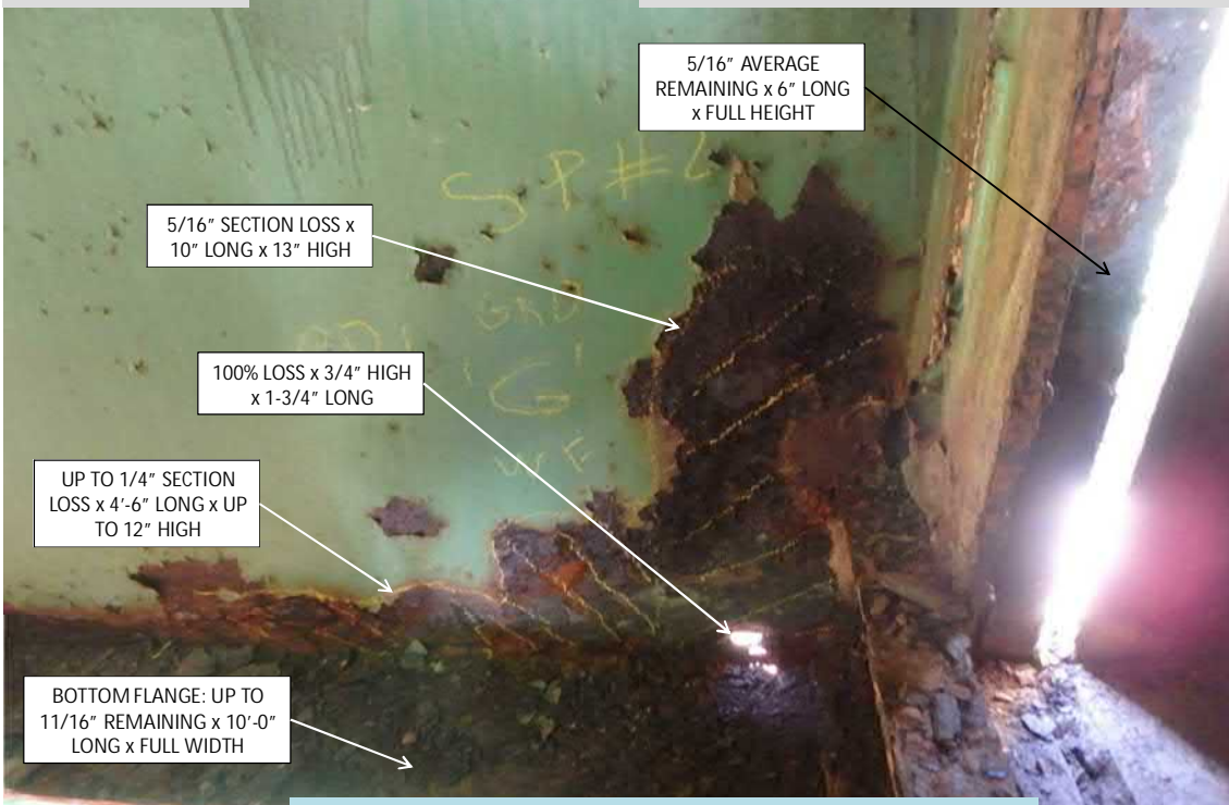
GIRDER 'G' – WEST FACE BRIDGE #067301 AT PIER 1 IN SPAN 2 (LOOKING EAST) 8/2/2018
