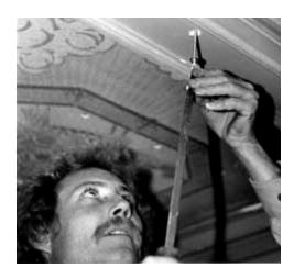
Where this ceiling was suffering from structural failure, the first step was to shore it up from below. Then, toggle bolts (seen here) were used to re-attach the plaster molding to the ceiling joists. Finally, the ceiling was patched, prior to restoring significant finishes. Photo: NPS files.
