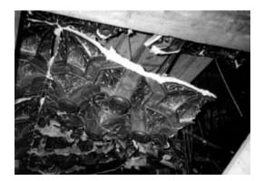
The Yiddish Arts Theater, New York City, c. 1920s. The concrete roof of this building had collapsed, damaging portions of the existing Moorish style coffered ceiling. The square coffer unit was easily identifiable and was removed to a casting shop for reproduction. Photo: David Flaharty.
