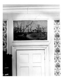
Settlement caused stress cracking through both flat wall and ornamental plaster. Repairs to the cornice molding involve chamfering the stress cracks to a "V groove," and patching with a mixture of gypsum and lime. Photo: Jack E. Boucher, HABS, NPS.
