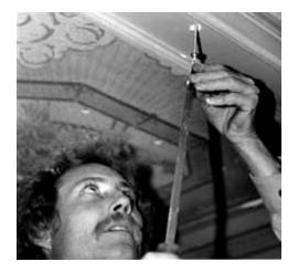
Where this ceiling was suffering from structural failure, the first step was to shore it up from below. Then, toggle bolts (seen here) were used to re-attach the plaster molding to the ceiling joists. Finally, the ceiling was patched, prior to restoring significant finishes. Photo: NPS files.
