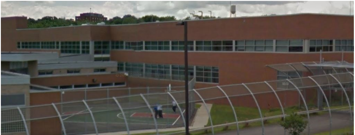
YDC Administration wing, east wall, storefront/curtain wall window systems This photograph is to be referred as detail 7/A102.
