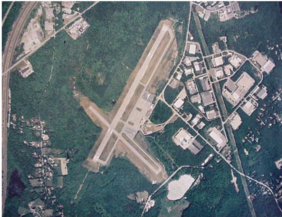
Figure 640-02(04) North Central Overhead Aerial
