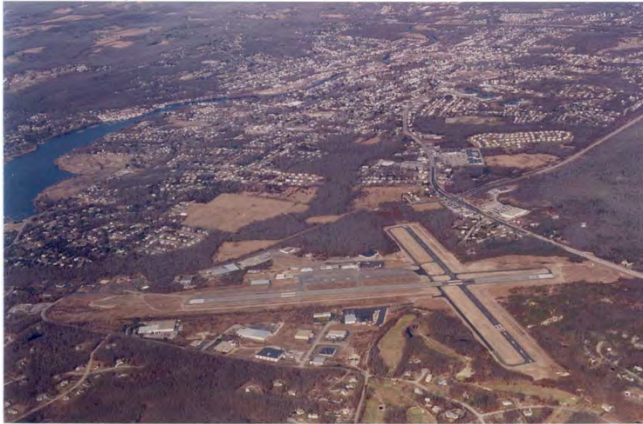
Figure 640-02(7) Westerly Overhead Aerial
